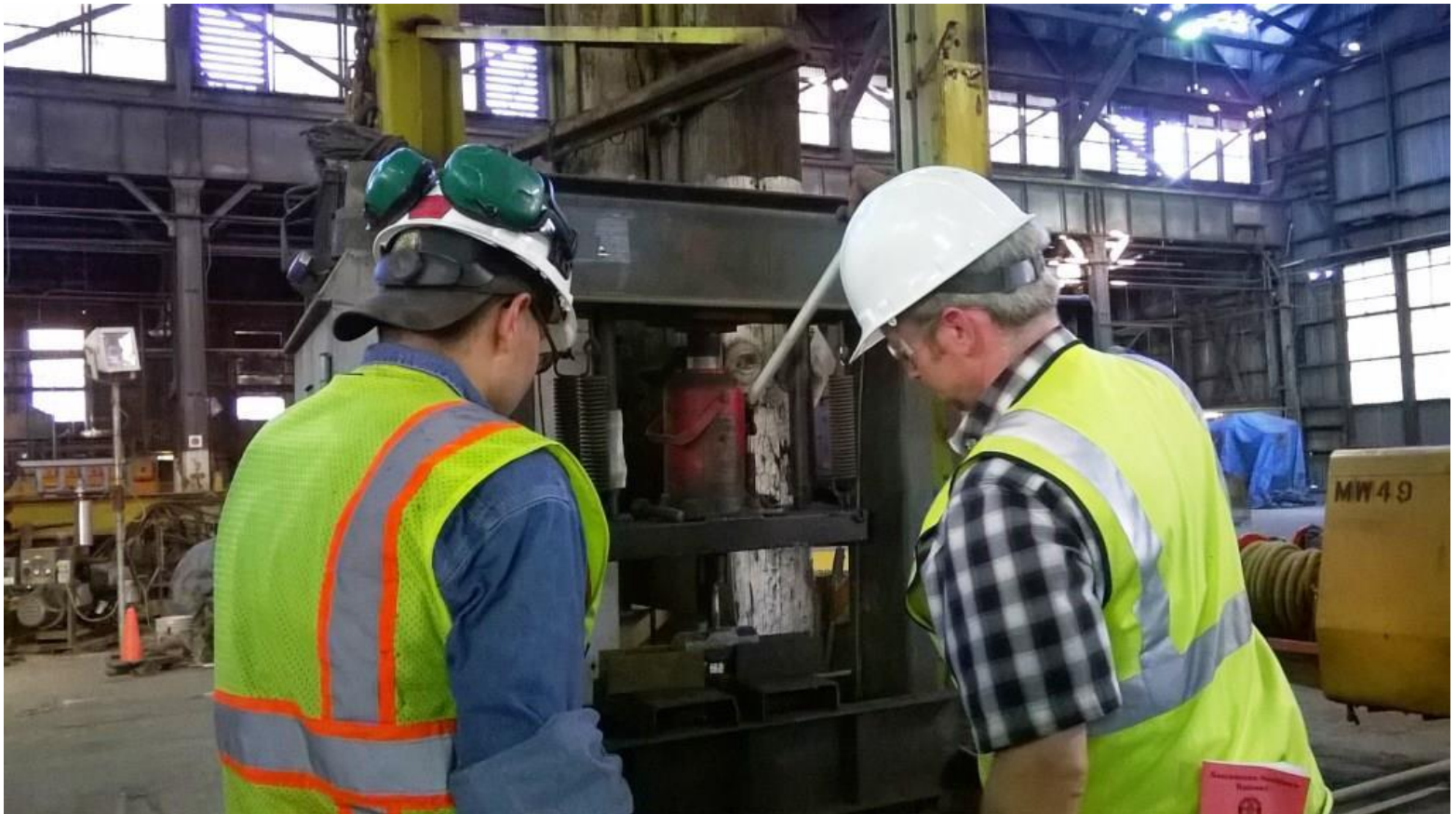
Kyle and Kevin work on replacing broken sledge-hammer handles
