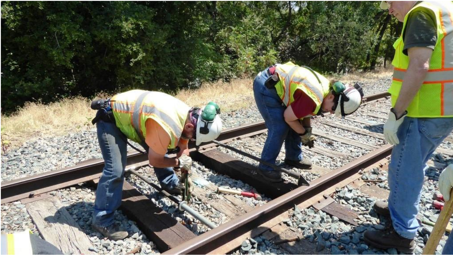
Joe and Heather use the rail spreader and track-gauge to re-gauge the track
