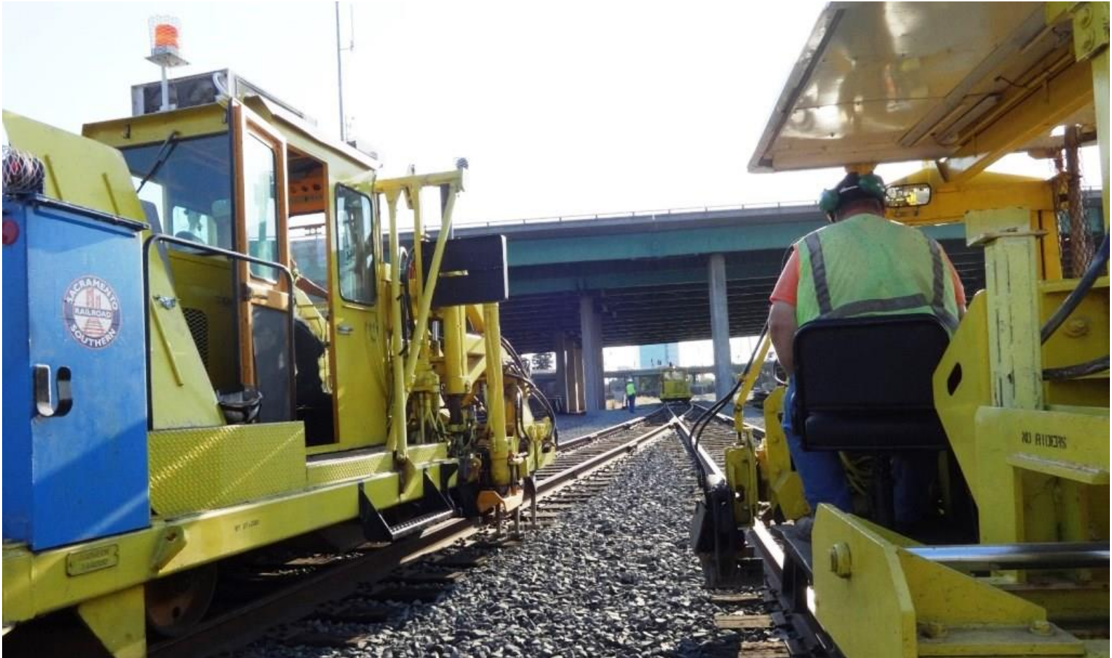
The tamper and the Jackson 125 are switched-out
